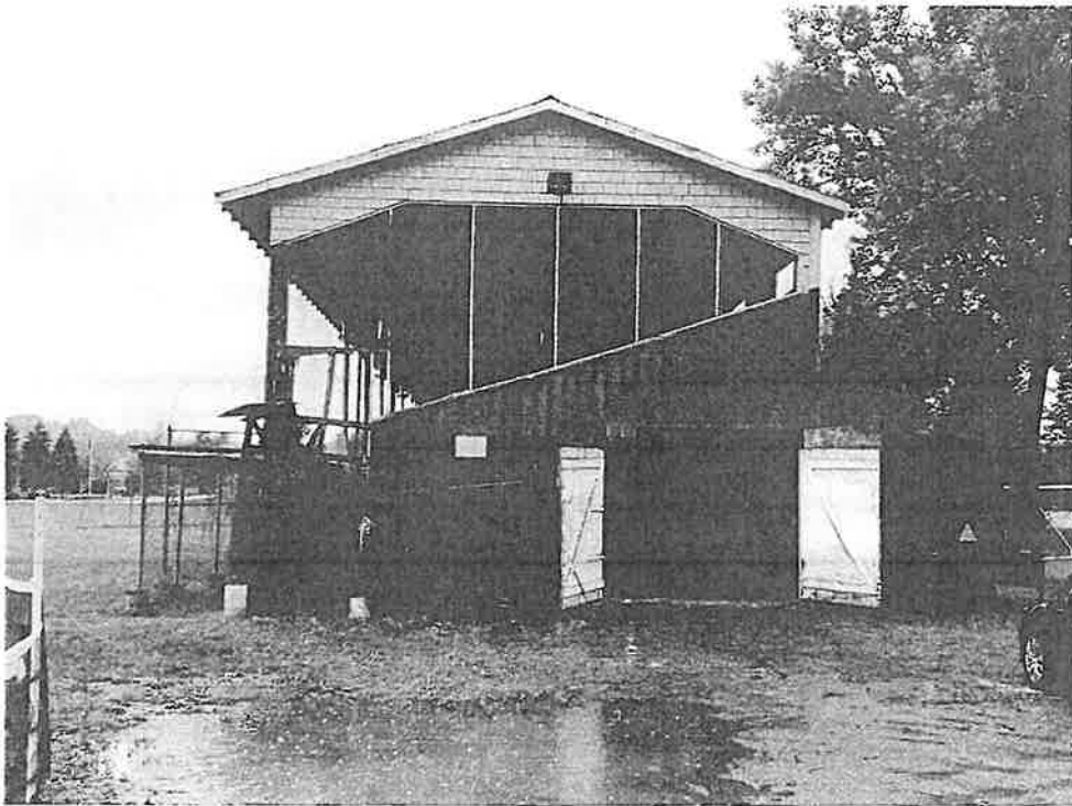
Grandstand - Side View Underneath Storage - Looking South
